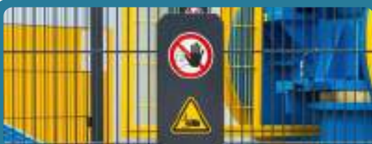
Safety Machinery Risk Assessment di Pabrik bahan Bangunan – Gresik
